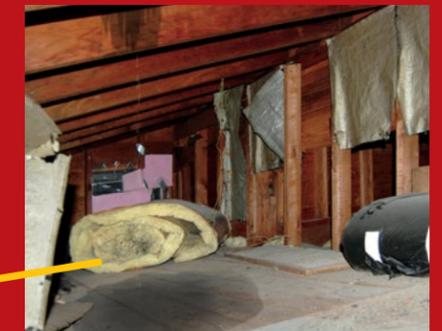
■ **Leakage in attic after driving rain.** Possible causes: Leaky or inadequate shingle underlayment; deteriorated flashing.
