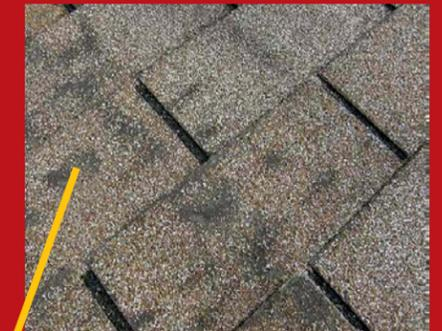
■ **Dark, "dirty-looking" areas on your roof.** Possible cause: Loss of granules due to age of shingles.
