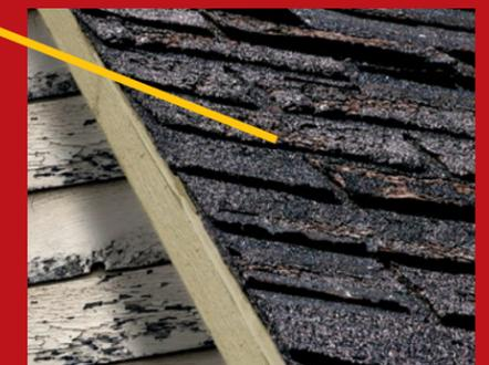
■ **Roof shingle, sheathing, and siding decay.** Possible cause: Poor attic ventilation.
