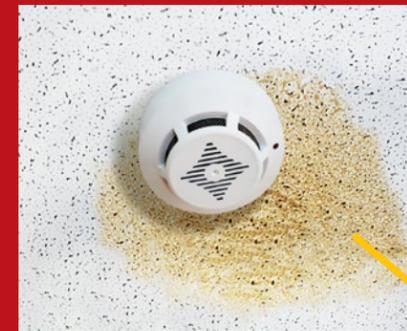
■ **Stains on interior ceilings and walls or mold and mildew growth.** Possible causes: Inadequate or faulty shingle underlayment allowing leakage, or inadequate ventilation.
