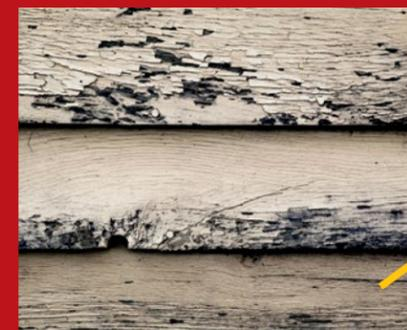
■ **Blistering and/or peeling of outside paint.** Possible cause: Excessive moisture or high humidity due to poor attic ventilation.
